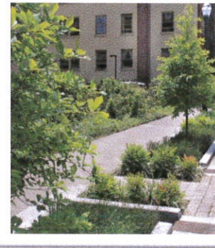
Stormwater planters (left) manage flow from impervious surfaces, allowing stormwater to infiltrate into the ground instead of the sewer system. The vegetation also filters pollution and reduces temperature. Photo: Oregon Environmental Services
