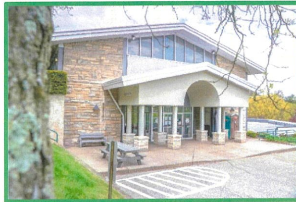
Whitehall Borough Building 100 Borough Park Drive Pittsburgh PA 15236
